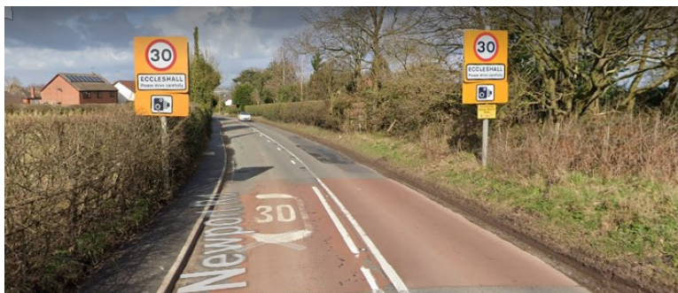
Newport Road, Eccleshall, where the pavements have received an innovative new compound as part of a surface dressing undertaken in March 2022
